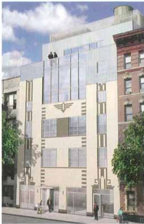
ABR's new 30,000 sf Medical facility at 429 East 75th St.
